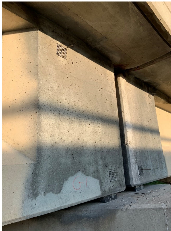
Figure 2 – Metalized Coating on Exterior Girder Ends
