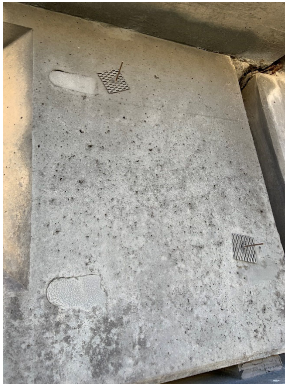
Figure 1 – Metalized Coating on Exterior Girder Ends
