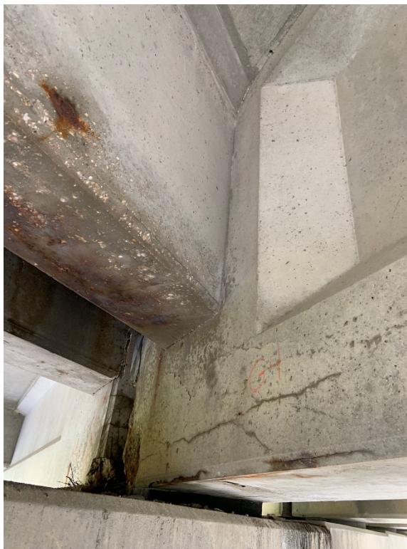
Figure 12: Cracked GE Bottom, G4 - SB Structure, Span 3, at Pier 3
