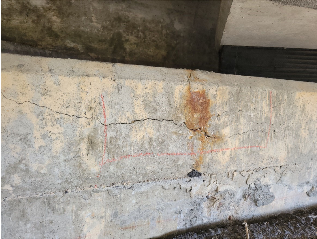
Figure 4 – Delamination in NB North Abutment
