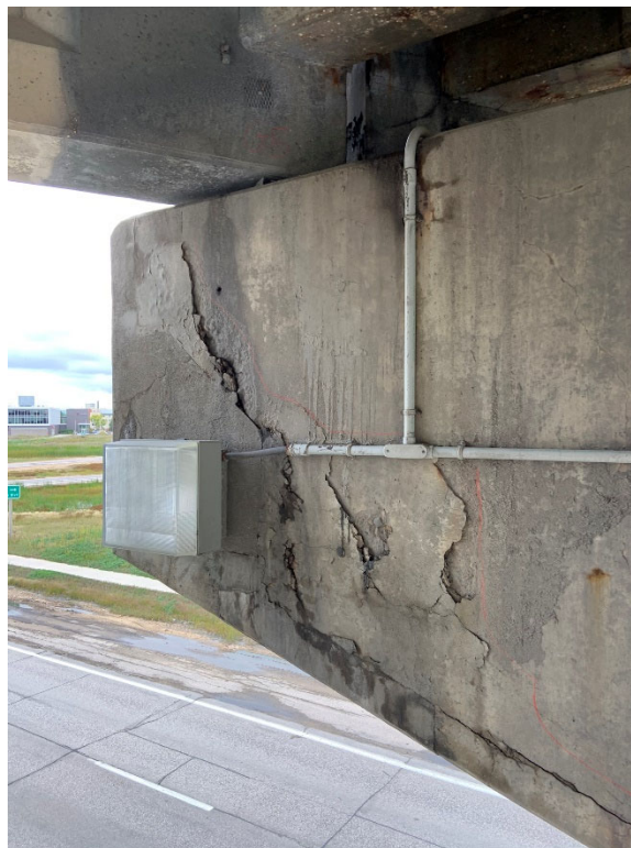
Figure 3 – Delamination in SB Pier 3 Hammerhead
