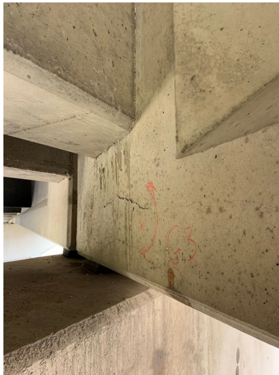
Figure 12: Delaminated GE, G3 – SB Structure, Span 1, at Pier 1
