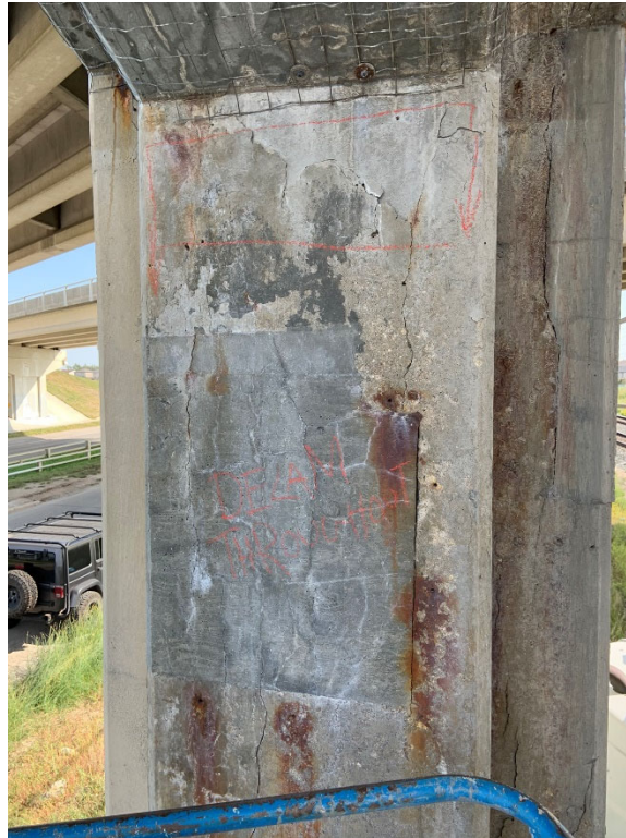
Figure 2 – Delamination in SB Pier 2 Ends
