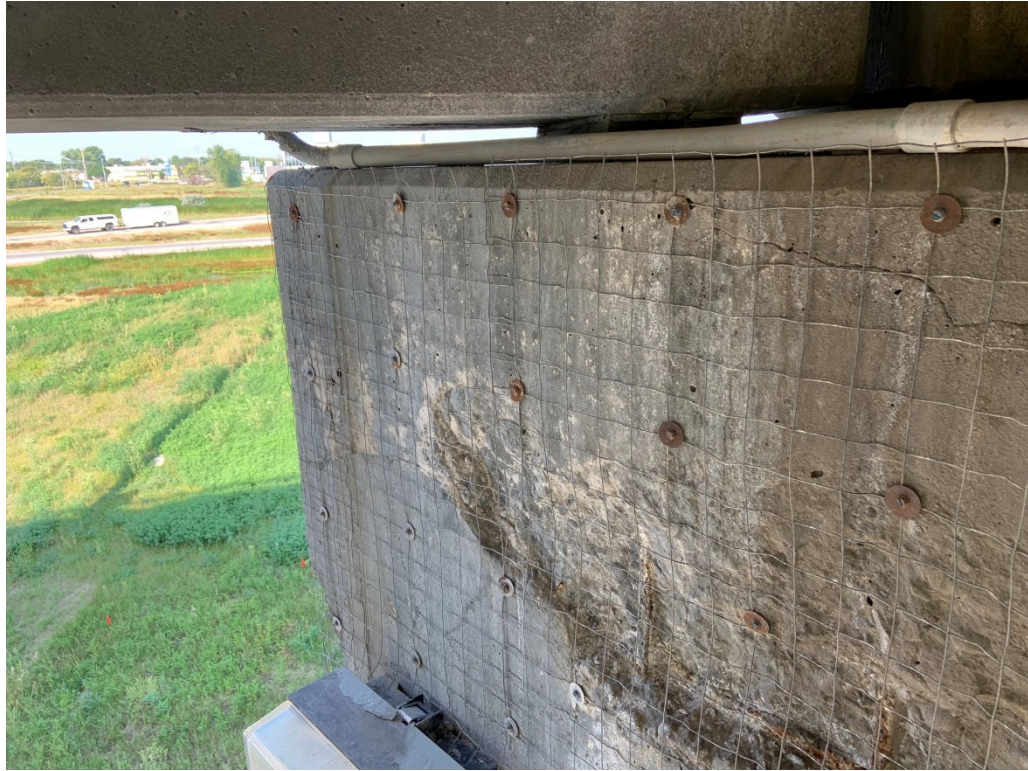
Figure 4 – Containment Meshing on Pier Hammerheads
