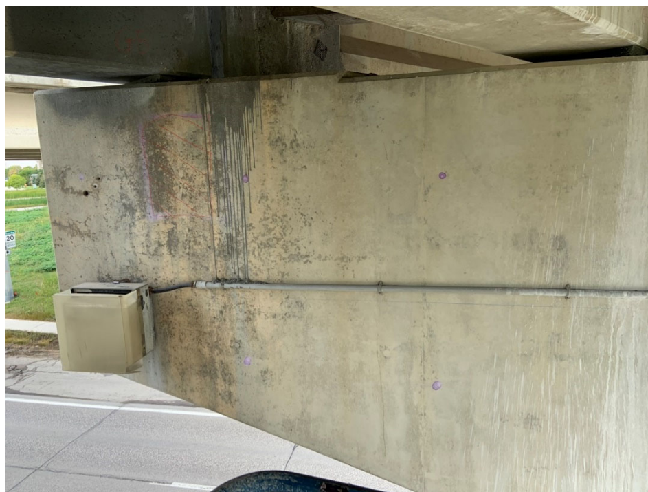
Figure 1 – Delamination in NB Pier 3 Hammerhead
