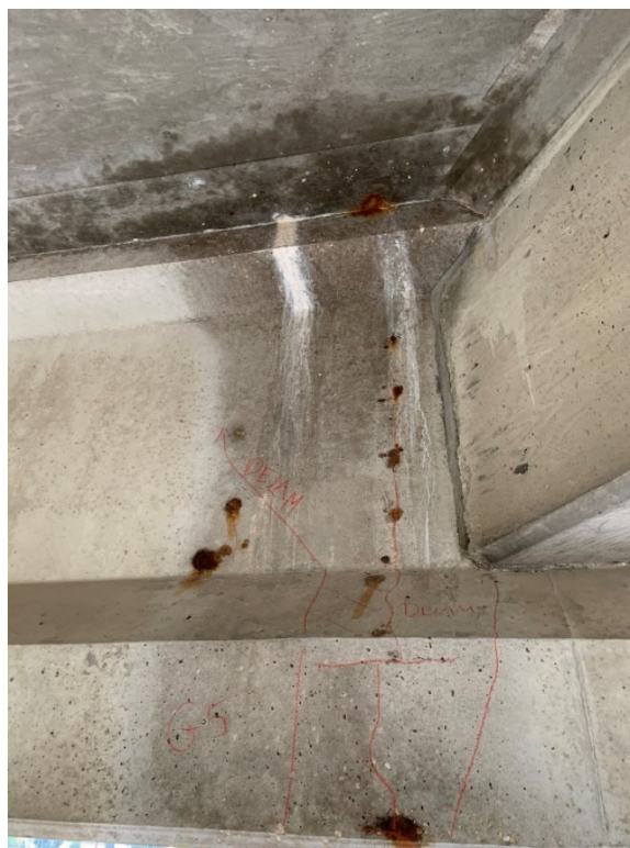
Figure 12: G5 Full Height Delamination (600mm wide) NB Structure, Span 4, between Pier 3 and South Diaphragm
