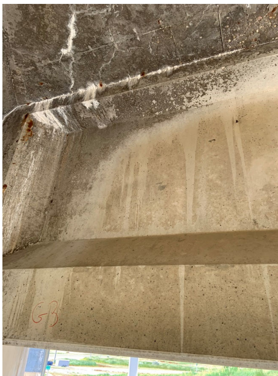
Figure 12: Surface Scaling Found at Various Locations
